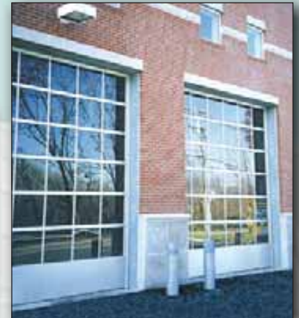
Milford Fire Dept., Milford, MA Installed by Door Systems, Framingham, MA
